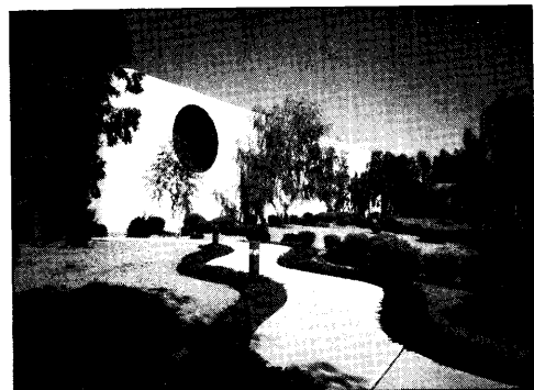
Tempe, Arizona: New 170,000-square-foot wafer fabrication facility.
